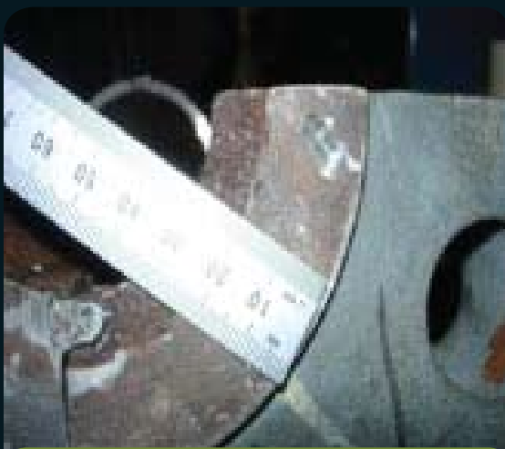
Typical Corrosion Pattern
